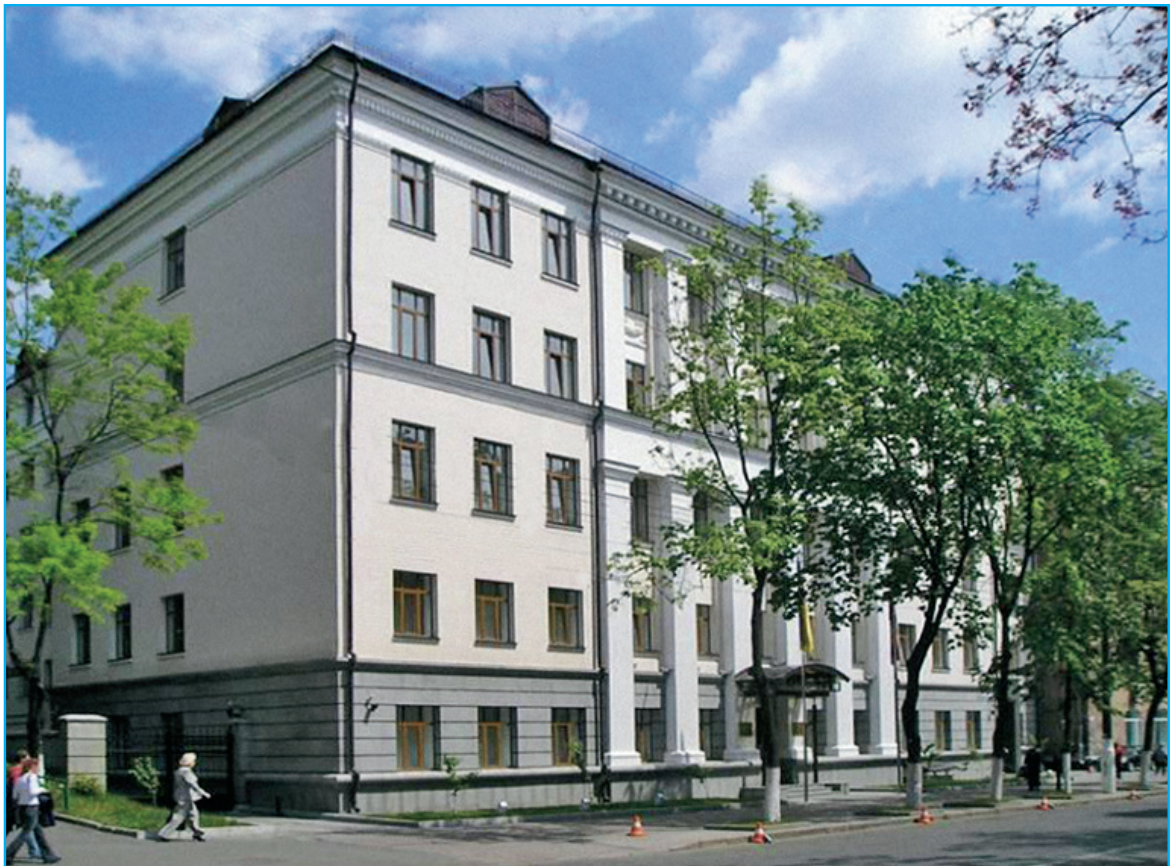
Pic. 1.2. Building of the SFMS
